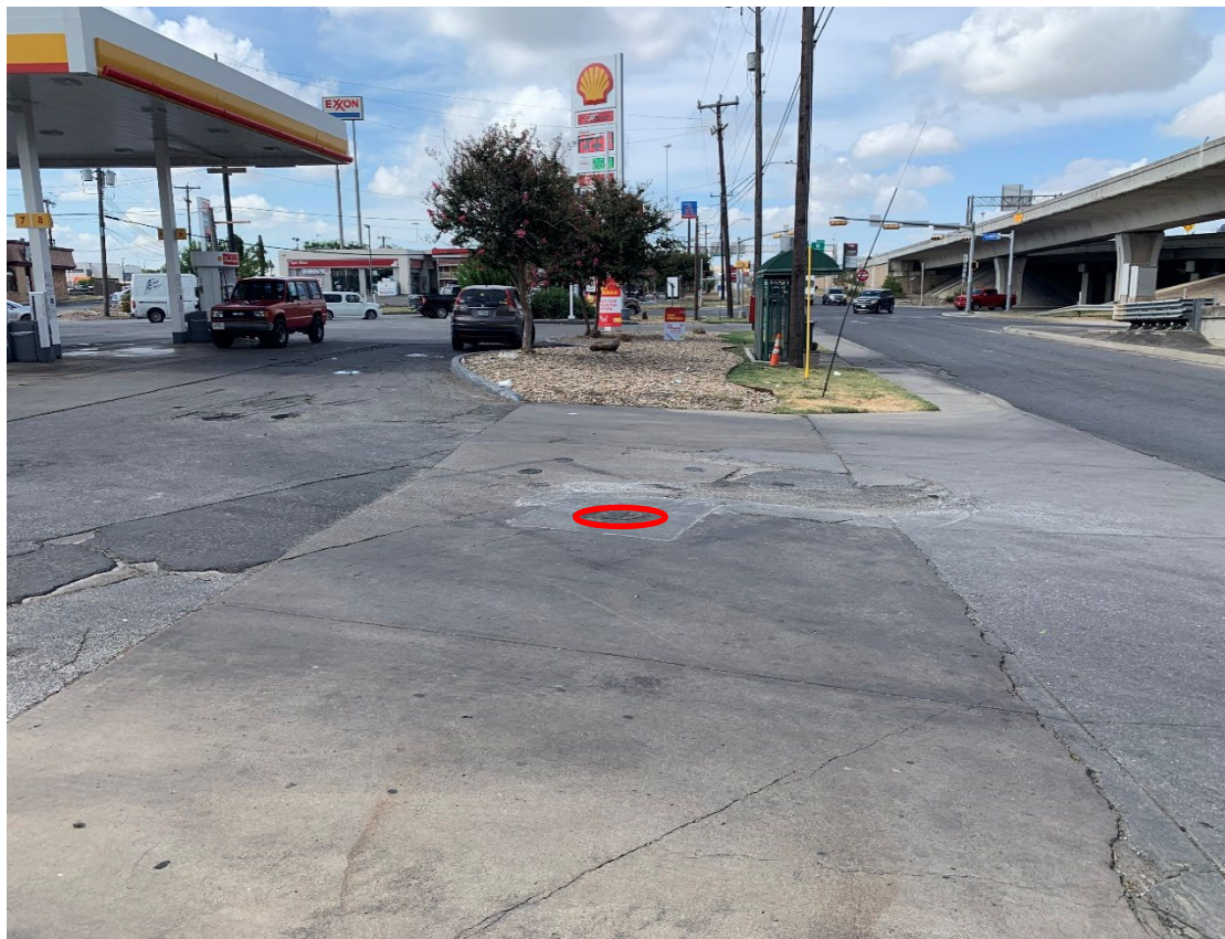
Existing upstream MH #38099 within Shell driveway
